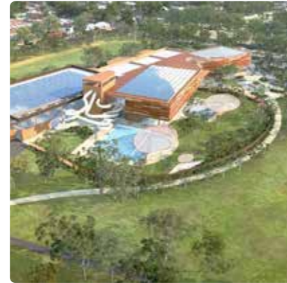
Adelaide Aquatic Centre, South Australian Government Under construction – opening summer 2025-26
