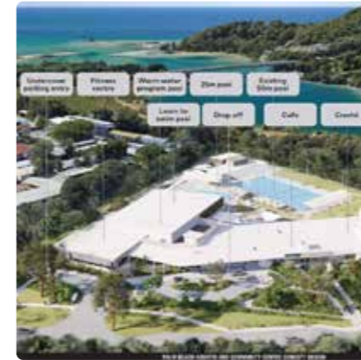
Palm Beach Aquatic and Community Centre, City of Gold Coast Stage two under construction – opening 2024
